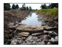
solutions are construction of riffles to slow the water (pictured), use of rock on the shoreline, tiering the side of channel to provide a natural high-flow bank, and underground piping (low-flow pipe).
