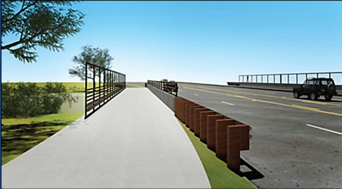
Five-lane bridge; 14-foot shared path on north side; 6-foot sidewalk on south side.
