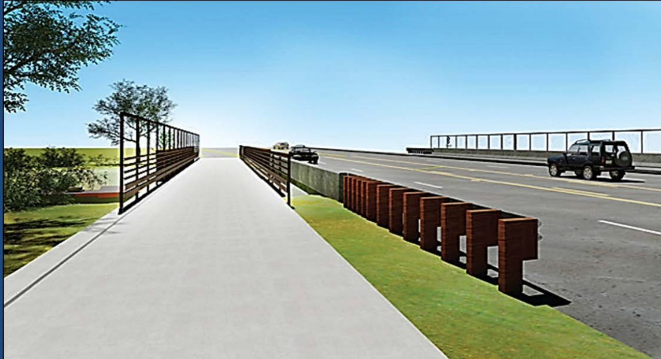
Five lane bridge 6-foot sidewalk on south; 2 nd bridge with 12-foot shared path on north side.
