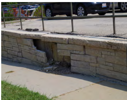
Above: A deteriorated retaining wall located on the west side of the Delta Communities property. (1316 East Empire Street)
