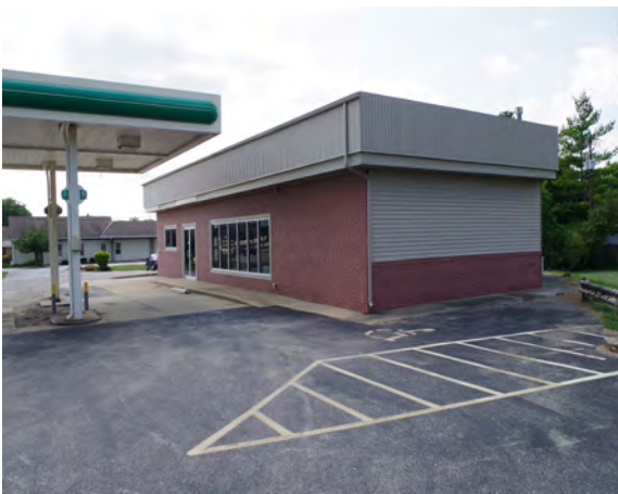
Left: A vacant former filling station. (1220 Towanda Avenue)
