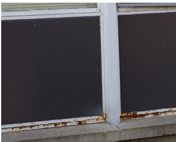
Left & Right: The windows sills at Bloomington High School are rusted and deteriorated. (1200 East Locust Street)
