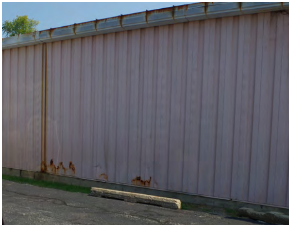
Left: The metal building, at the rear of this multi-tenant commercial building, is dented and the gutters and siding are rusted. (1328 East Empire Street)
