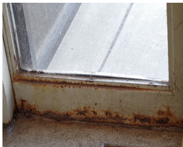
Left & Right: The windows sills at Bloomington High School are rusted and deteriorated. (1200 East Locust Street)
