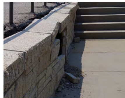
Above: A deteriorated retaining wall located on the west side of the Delta Communities property. (1316 East Empire Street)
