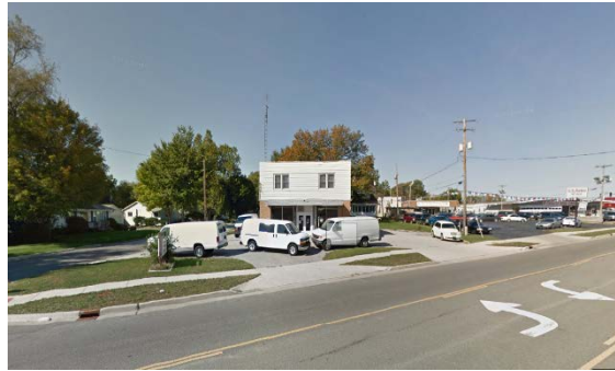
East view from Morrissey
