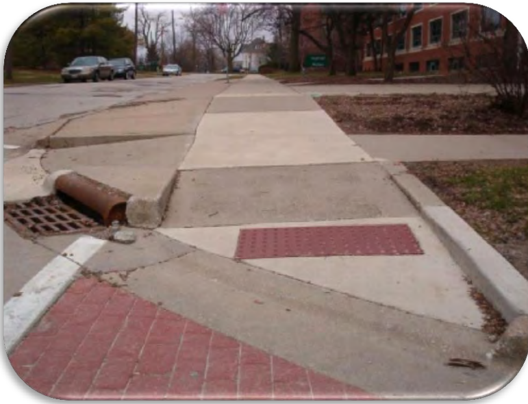
Type A: Ramps typically adjoin grassy areas, so curbs along the ramps themselves are necessary
