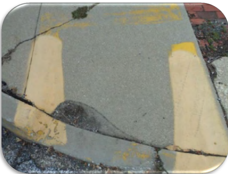
Type B: Ramps have side flares instead of curbs and usually are surrounded by concrete.
