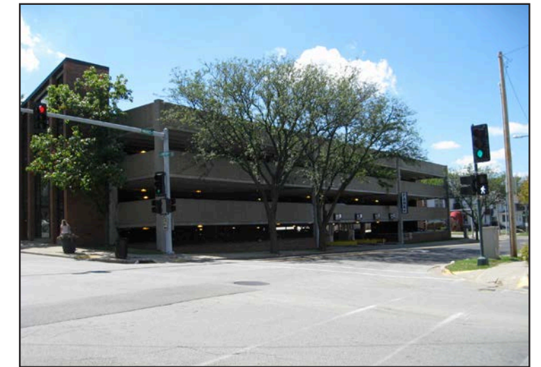
Market Street Public Parking Garage.
