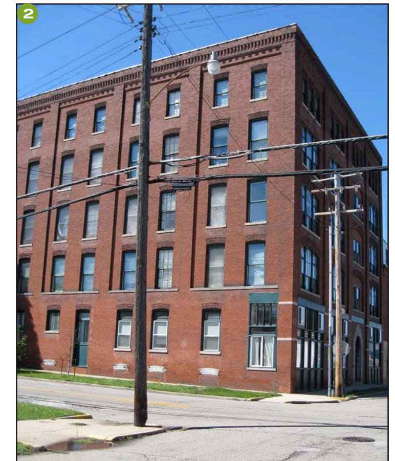
Figure I-10. The White Building typifies commercial and warehouse buildings of its time. The design featured numerous windows to let in light and air before buildings were wired for electricity.
