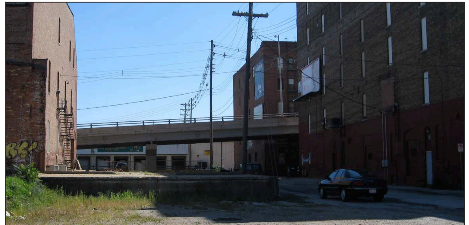
Figure III-10. The Main/Center overpass cuts through blocks of the Warehouse District, creating a sunken affect in the area.
