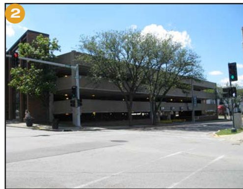
Market Street Parking Garage.
