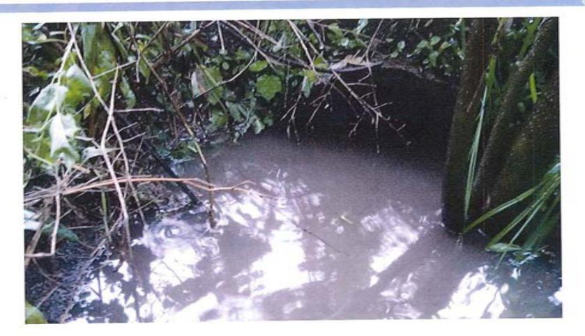
Location C output pipe nearly totally submerged during average rain event.
