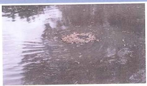
Location E street surface drains also fail to accept water when the swale volume is high.
