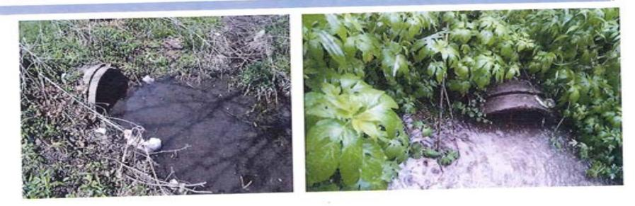
Swale water volume nearly totally submerges Cardinal Ridge output pipe D during an average rain event.
