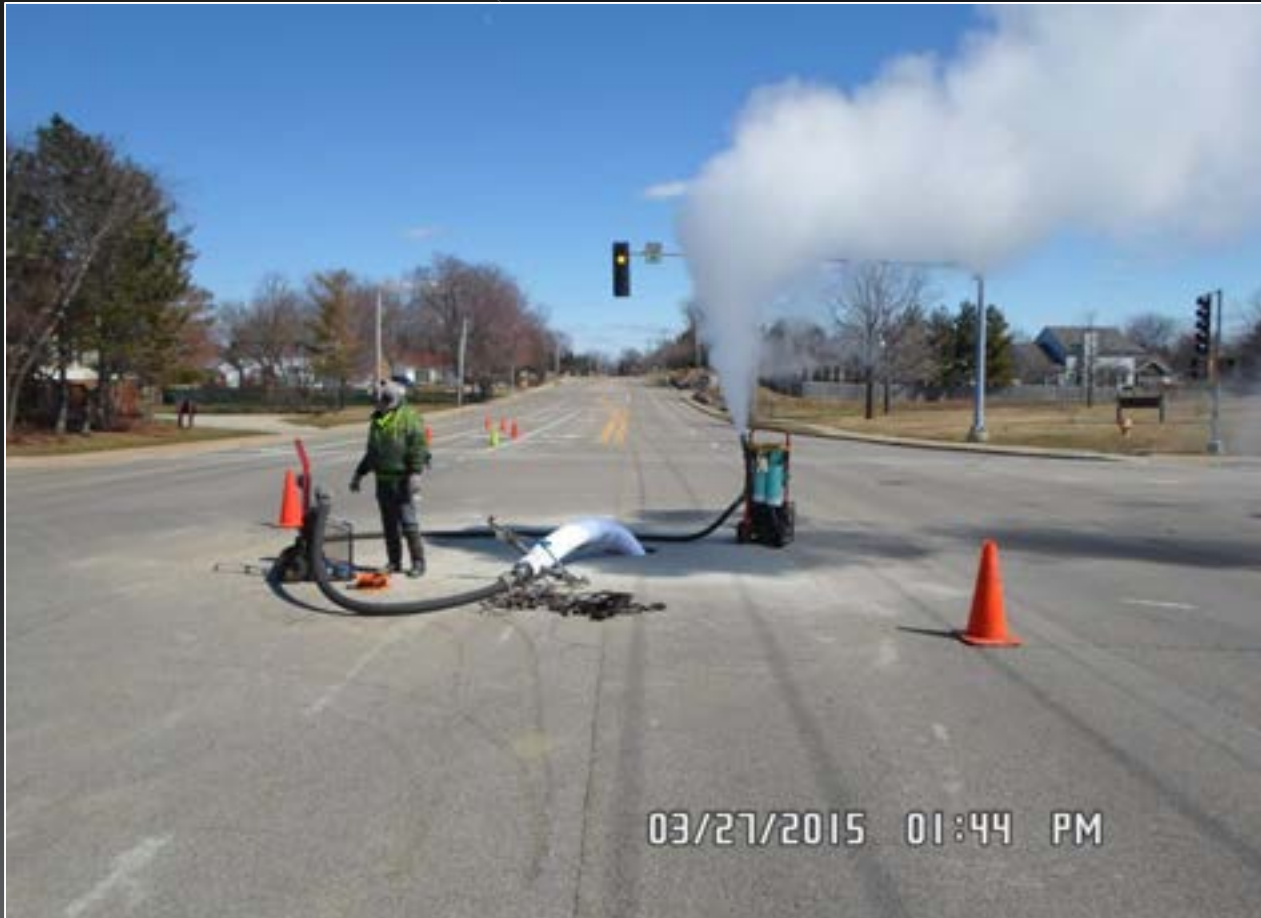
Above: East-side lining as part of an ongoing I/I pilot study.
