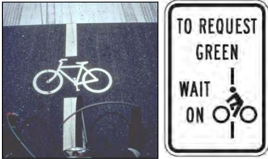
Figure 2.12. Signal activation marking and sign.
