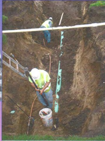
Crews replacing sewer & water services
