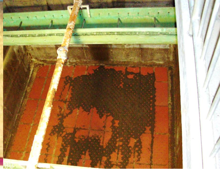
C. View looking into filter with media removed
