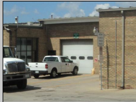
Office, 402 S. East Street
