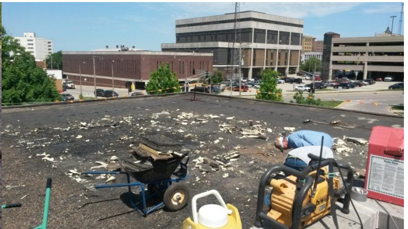
Clearing Roof Debris
