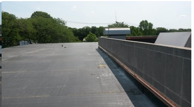
New roof Membrane & Flashing
