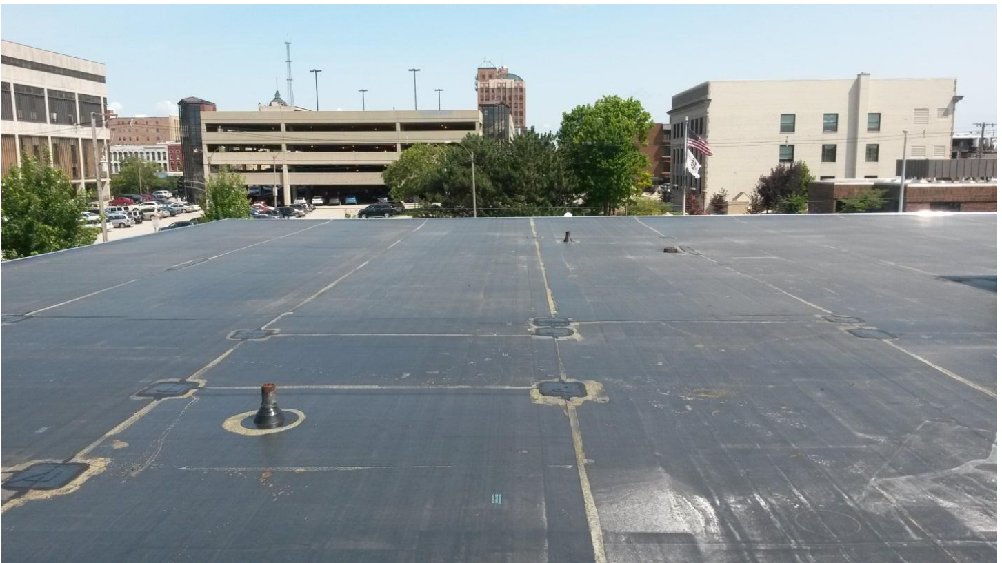
New Roof Membrane & Flashing
