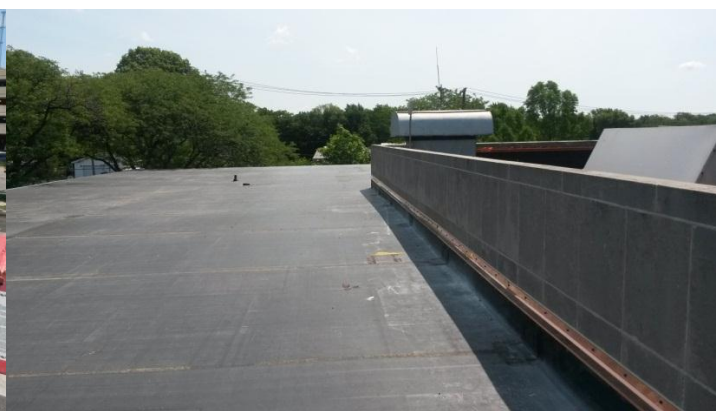
New Roof Membrane & Flashing
