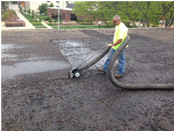
Vacuuming Aggregate Roofing Rock
