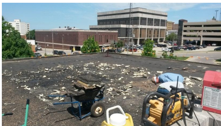
Clearing Roof Debris
