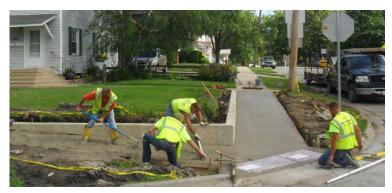
installation of retaining wall to keep the adjoining yard at grade. An ADA compliant ramp usually costs \$1,200 to install. This one cost \$4,200 because of the associated sidewalk and retaining wall installation.
