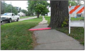
sidewalk around the tree, as there is ample space in the parkway, or it will use reinforced concrete for the sidewalk surface to bridge the flare of the tree and reduce the likelihood of
