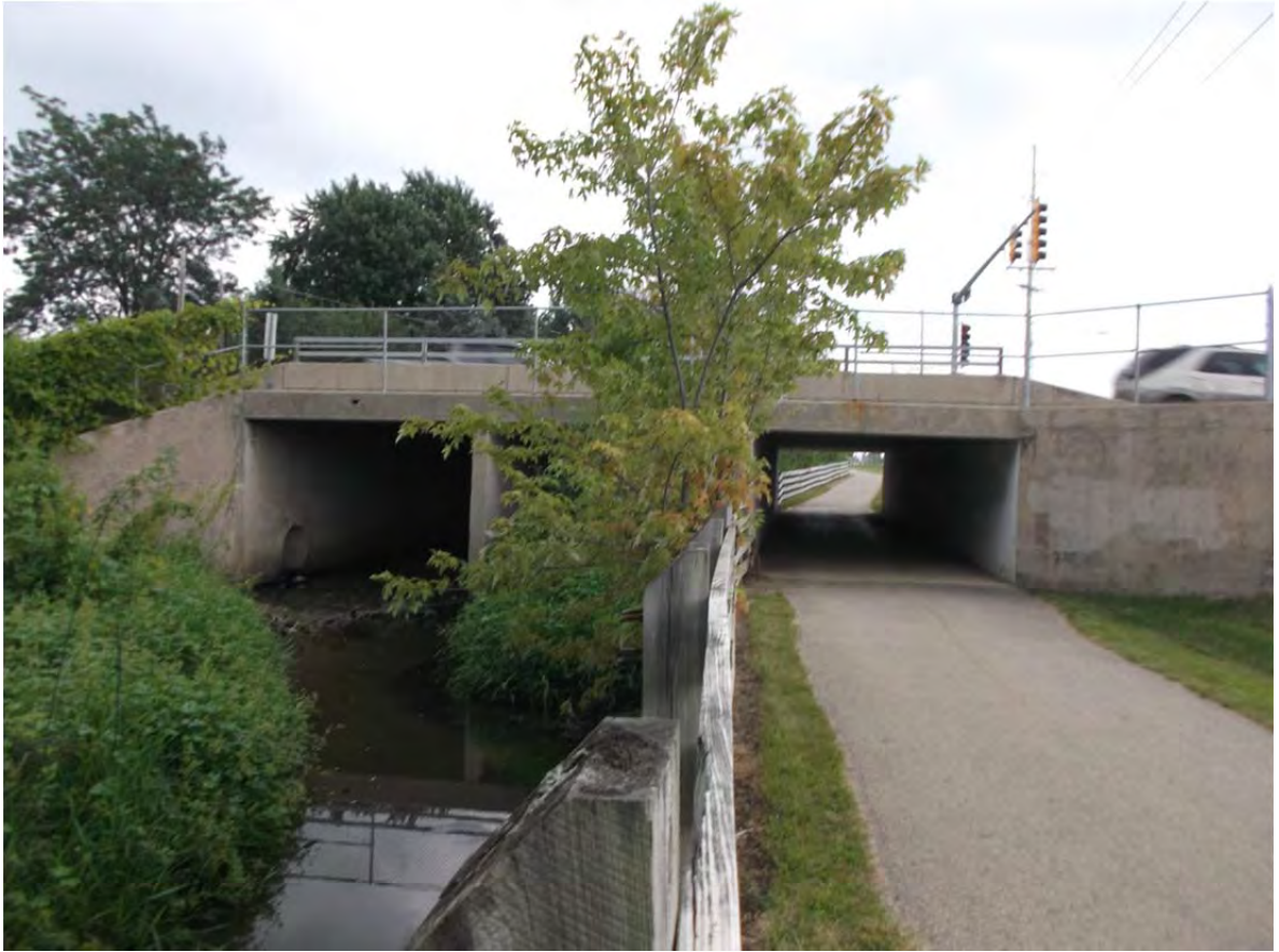
Hershey Road- Pedestrian Underpass / Drainage Structure at G.E. Road
