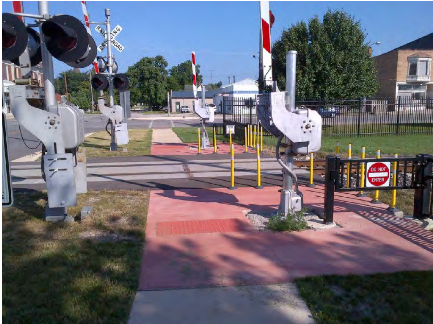
Typical pedestrian rail crossing installation
