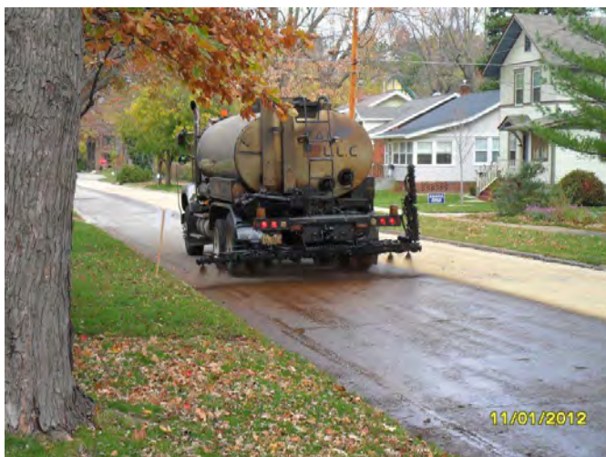
Figure 7 - Moore Street during application - other side is done
