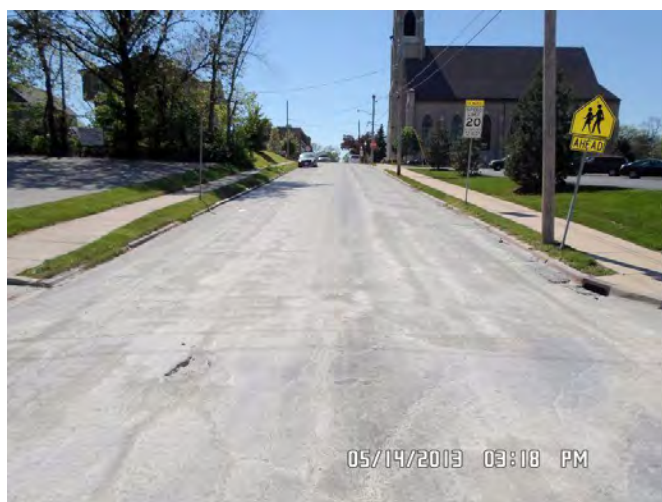
Figure 10- Jackson Street 9 days after CRF treatment
