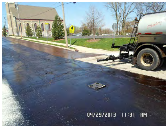
Figure 9 - CRF just applied to north side of Jackson Street. South side has cured to black color after 15 minutes. Lime screenings on Oak Street are visible on left side of picture.
