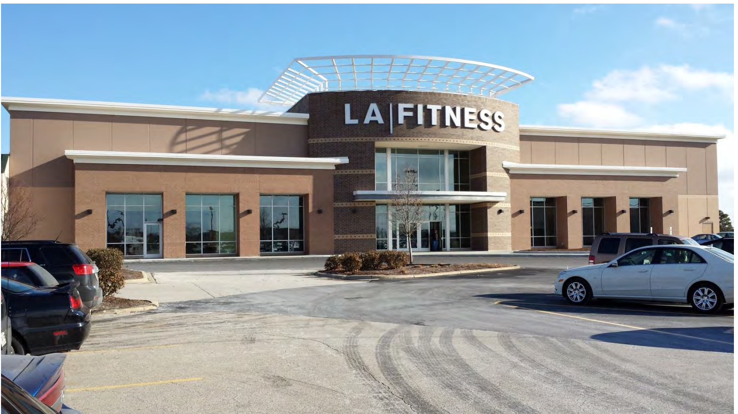
Recently completed LA Fitness located at 2103 North Veterans
