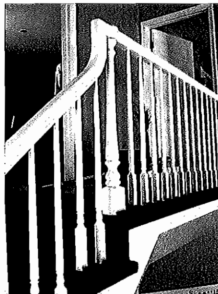
Transition from handrail to guard
