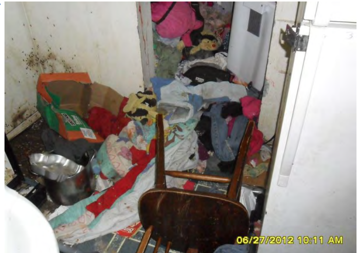
Interior property maintenance problems. Note the roaches on the walls.
