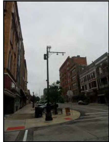
Figure 7: Camera & Wireless Access Point Pole Example
