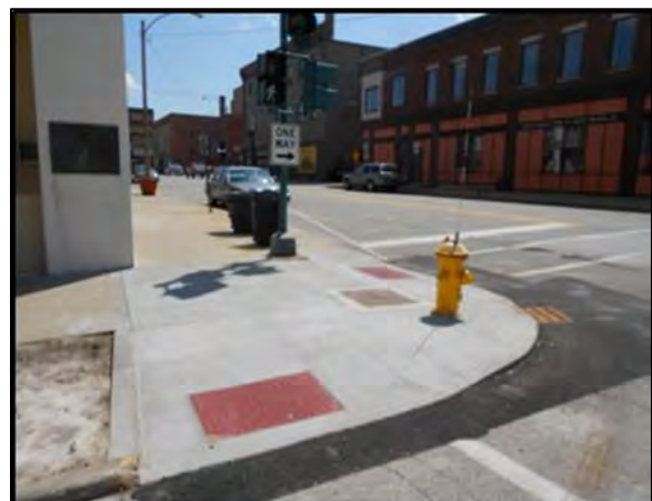
Figure 6: Example of Completed Inlet Repair Work
