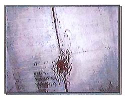
Several of the steel connections between the precast beams and columns have begun to rust. Some of these connections have grout covers over the steel that are cracked and spalled.
