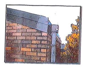
7. The concrete framing and brick wall outside the Northeast stairwell doorway on the First through Third Levels was wet with rainwater. The exact location of the water infiltration could not be determined, but the following issues were noted: rainwater is leaking under the door into the Fourth Level of the Northeast stairwell, and the sealant at the flashing around the Fourth Level door and walls appears to be cracked and brittle, in some locations.
