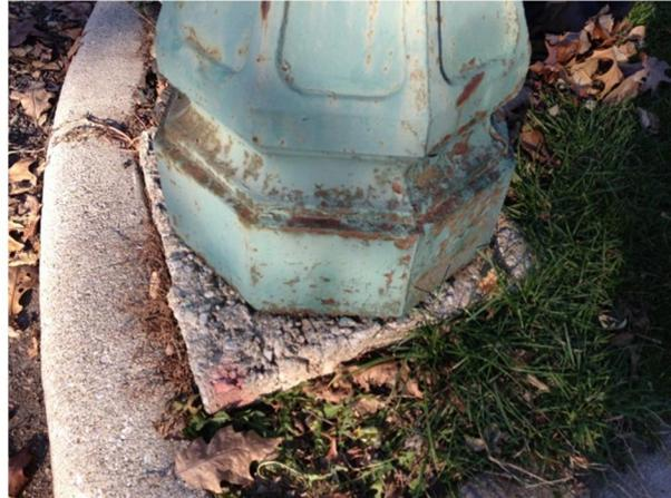
**Figure 3** - *An existing concrete foundation deteriorating beneath a pole base.*
