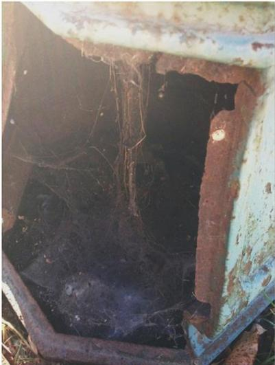
**Figure 4** – Interior deterioration shown in one of the 12 decorative pole bases.
