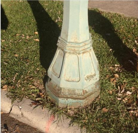
**Figure 2** - *An existing pole base foundation shown sunk into the soil allowing increased weathering around the base.*
