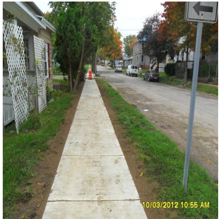
After installation of sidewalk on Clayton Street
