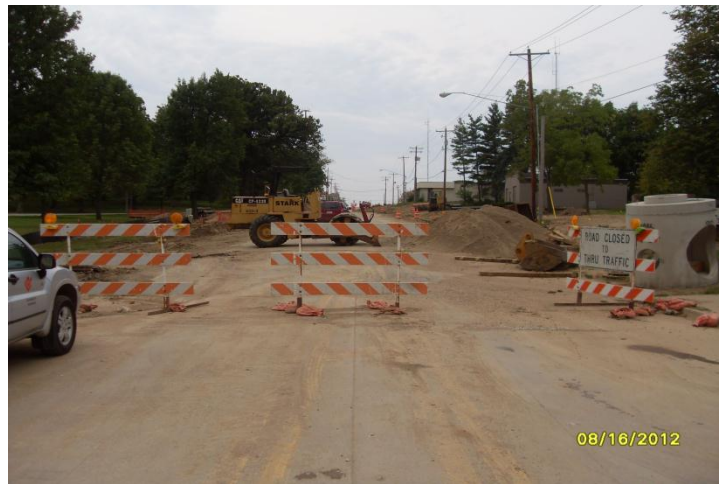
Morris Avenue During Construction
