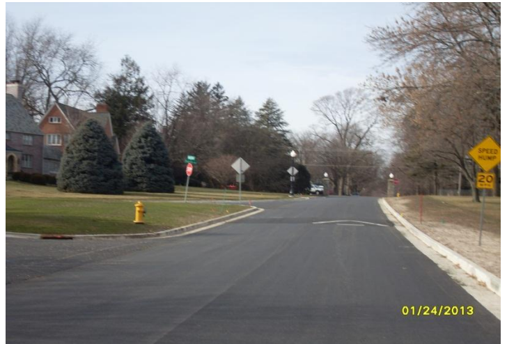
Country Club Entrance- After Construction
