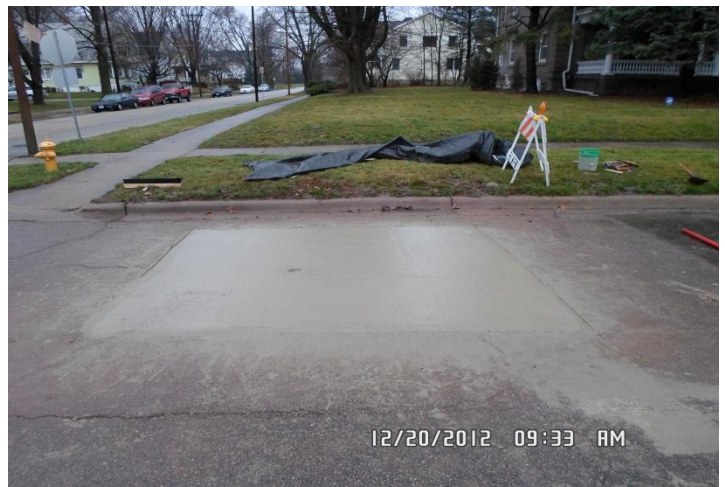
Completed Water Ditch Repair
