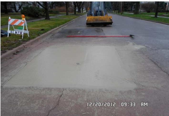
Completed Water Ditch Repair
