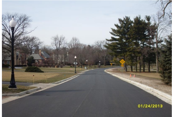
Country Club - After Construction
