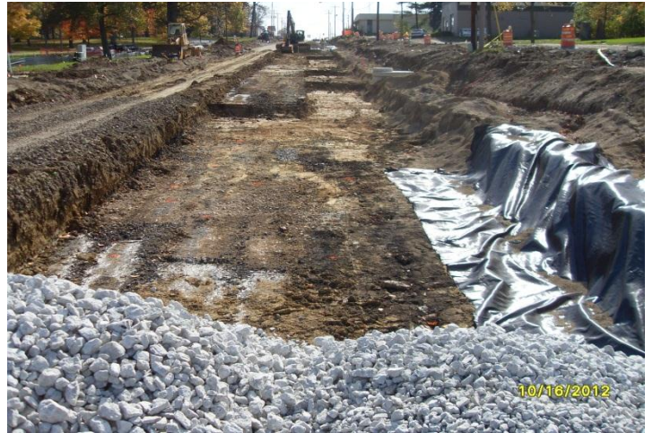
Morris Avenue During Construction
