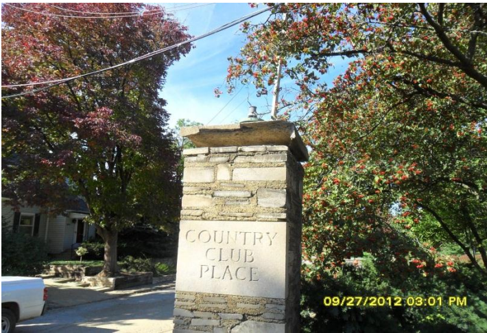
Pillar Before Construction
