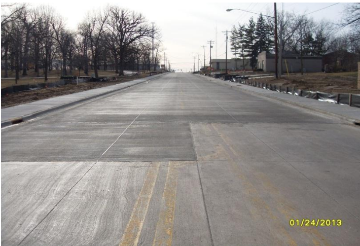
Morris Avenue After Construction
