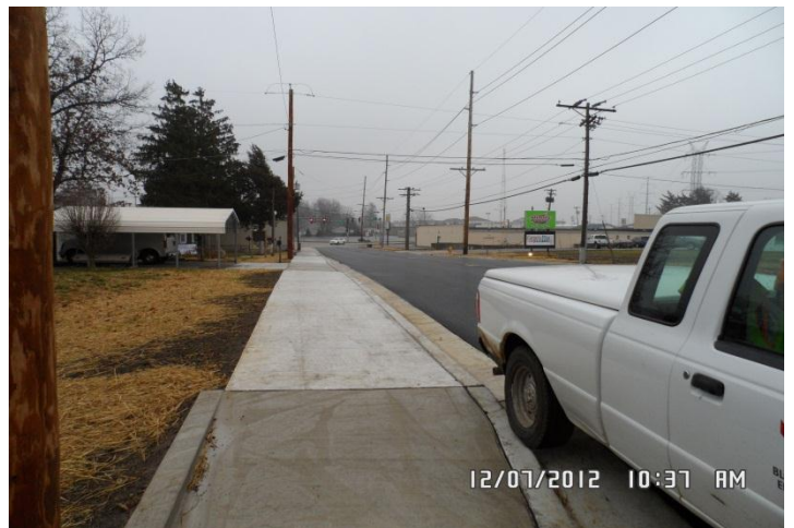
Lafayette After Construction
