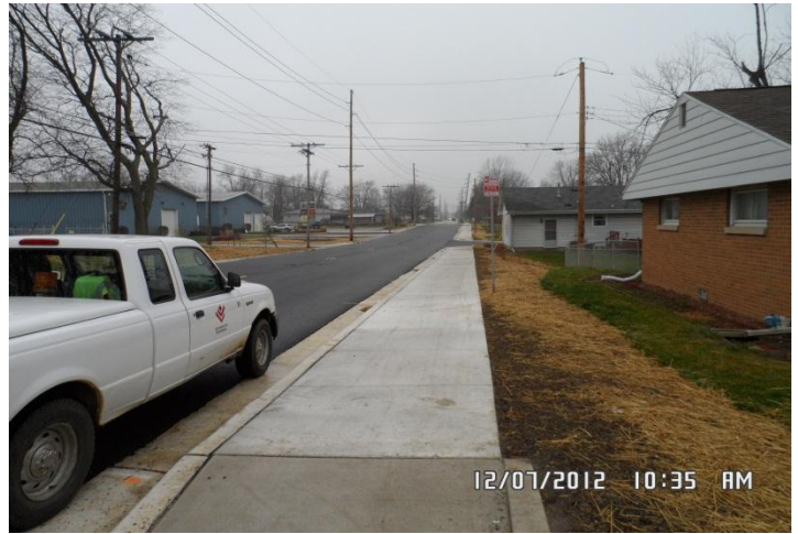
Lafayette After Construction
