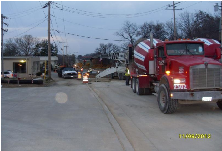
Morris Avenue During Construction
