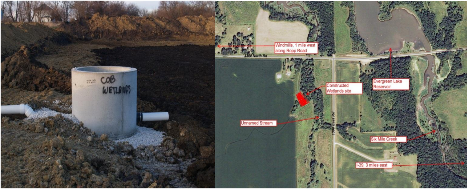
Evergreen Lake Reservoir Constructed Wetland Site
