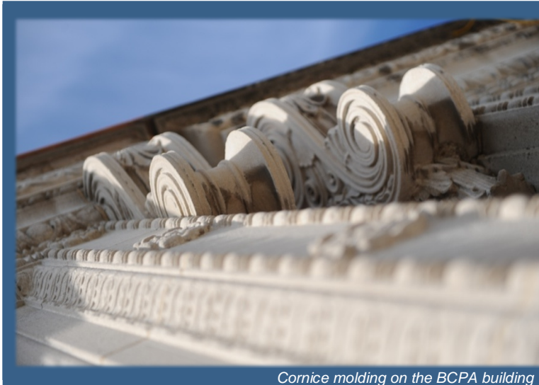
Cornice molding on the BCPA building
