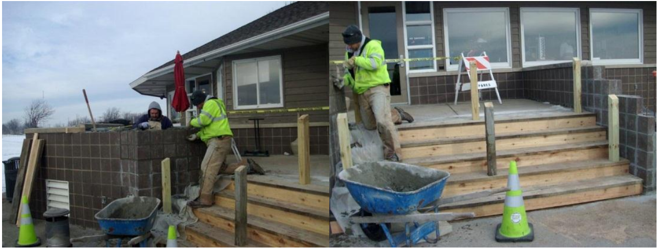
Staff working on the stairs at Prarie Vista Golf Course
