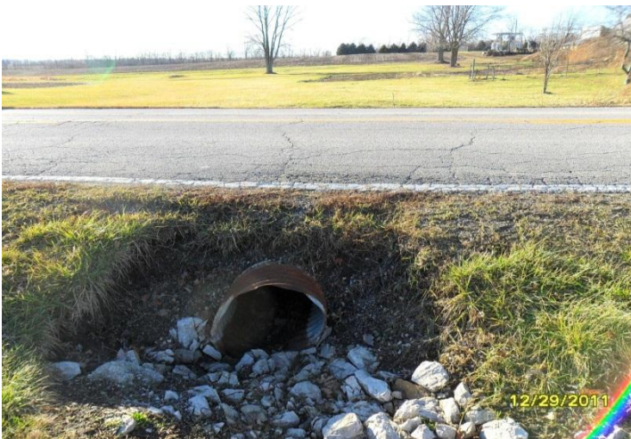
Morris Culvert Before
