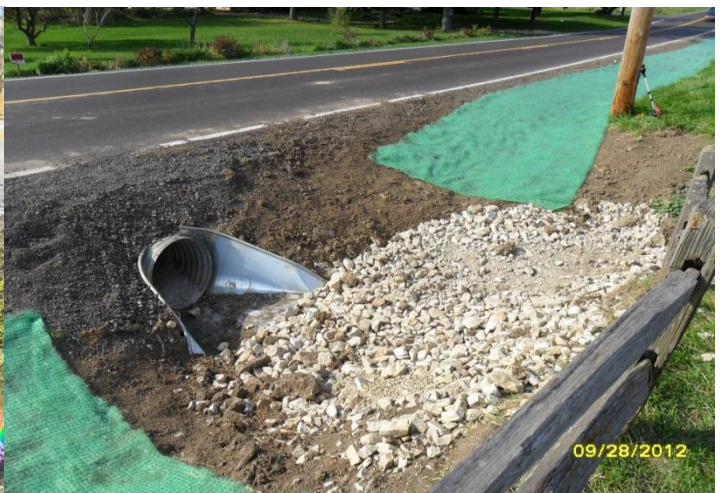
Morris Culvert After
