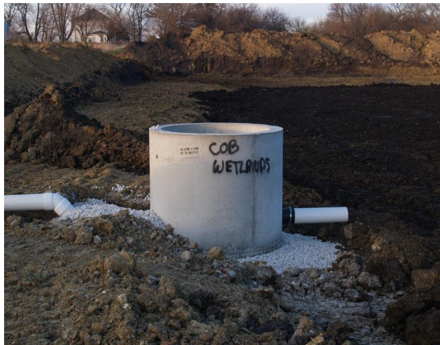
Wetland Inlet Structure Under Construction- Nov 2012
