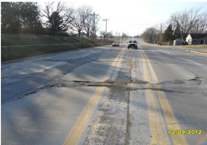
Lincoln Street East Before
