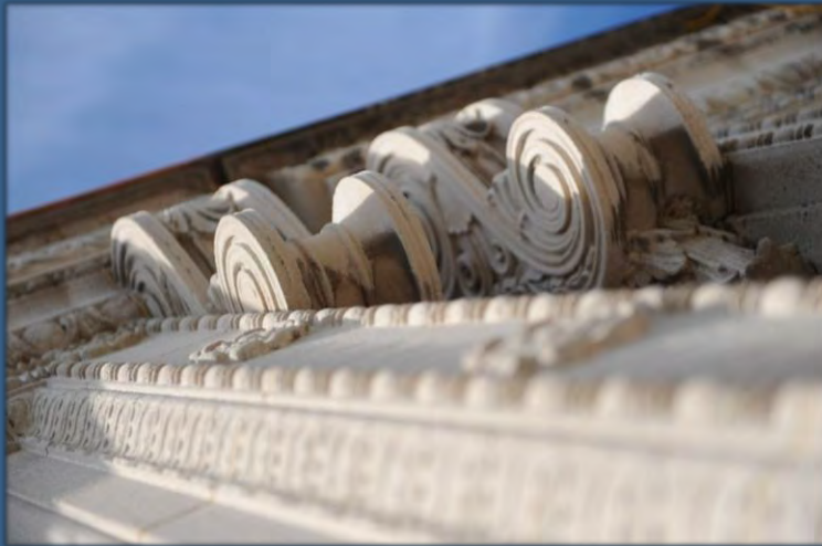
Cornice molding on the BCPA building
