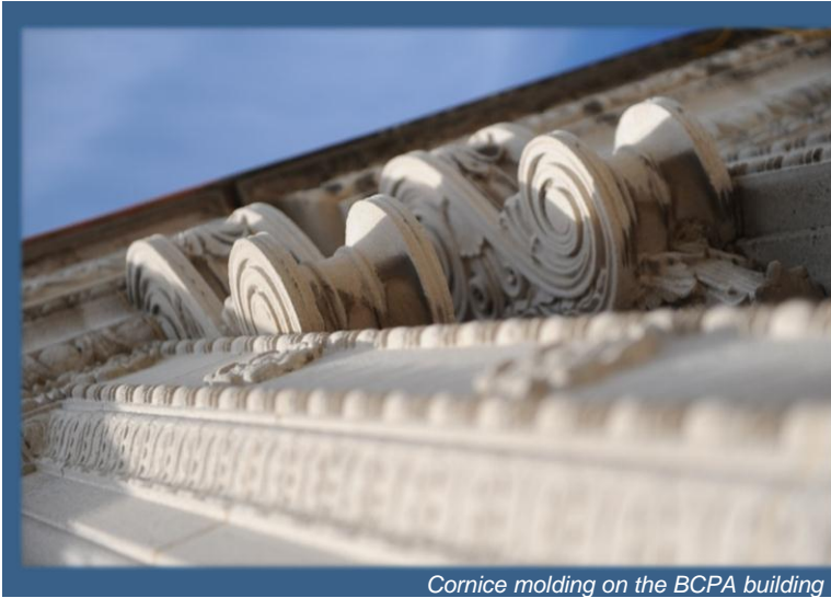
Cornice molding on the BCPA building
