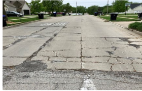
Old Jamestown Rd
