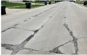
Old Jamestown Rd
