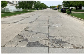
Old Jamestown Rd
