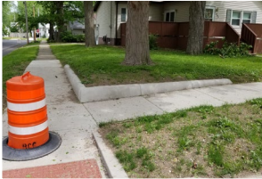
FY25 Street, Sidewalk, & Alley Maintenance
