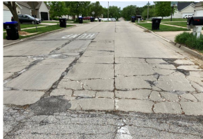
FY25 Concrete Streets
