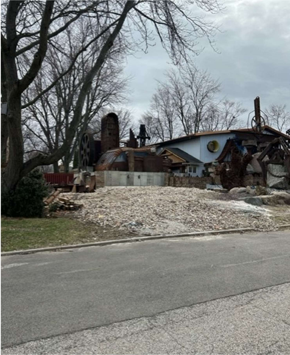
Attachment 3 - Ground-Level Views (from Garling Drive)
