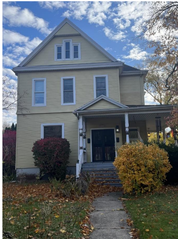
Above: The subject property at 1001 N. Evans Street
