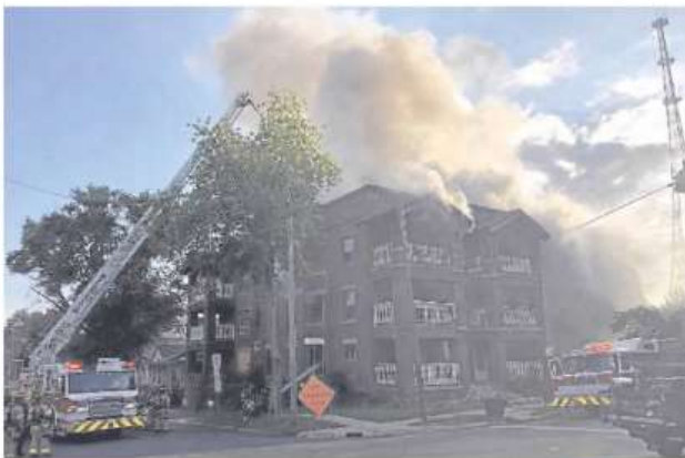
COURTESY OF THE BLOOMINGTON FIRE DEPARTMENT The Bloomington Fire Department responded to a structure fire Wednesday morning at Lee and Market streets in Bloomington.
