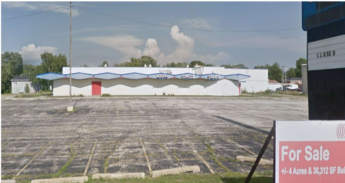
Above: The subject property at 1225 Holiday Drive
