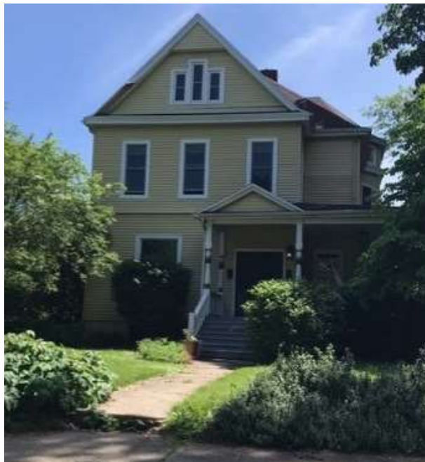
Above: The subject property at 1001 N N Evans Street
