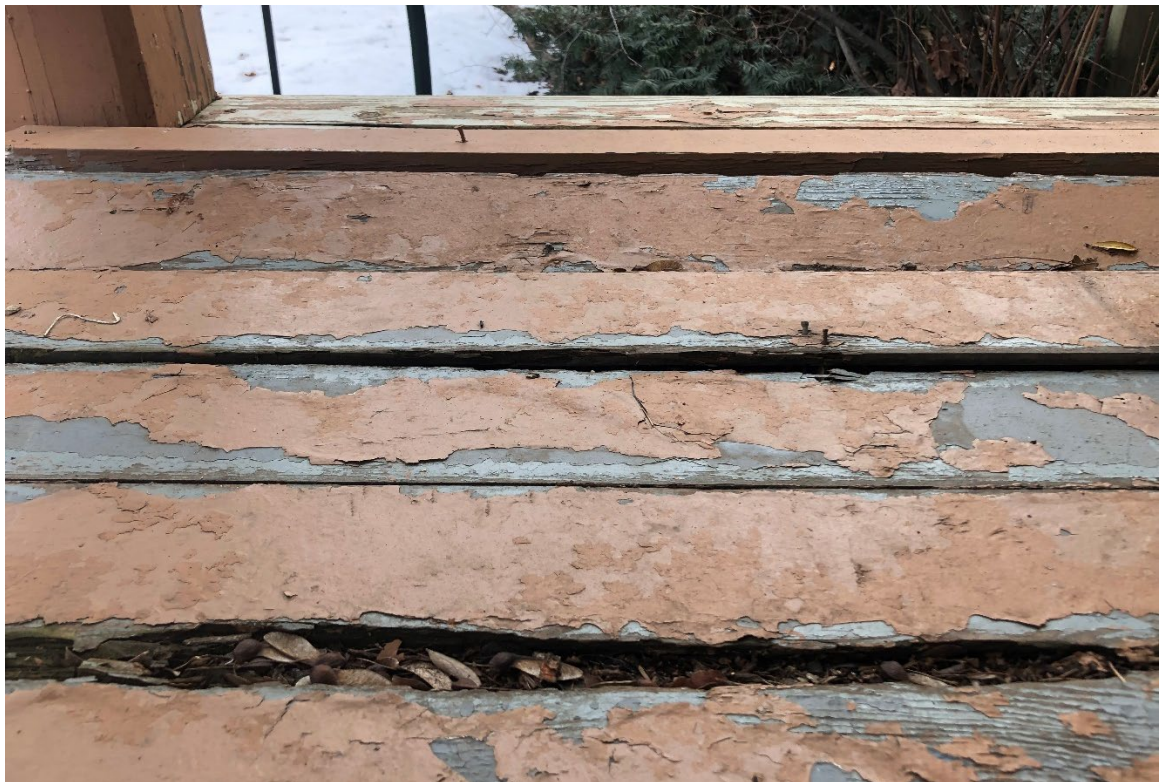
Wear and buckling to the deck boards.
