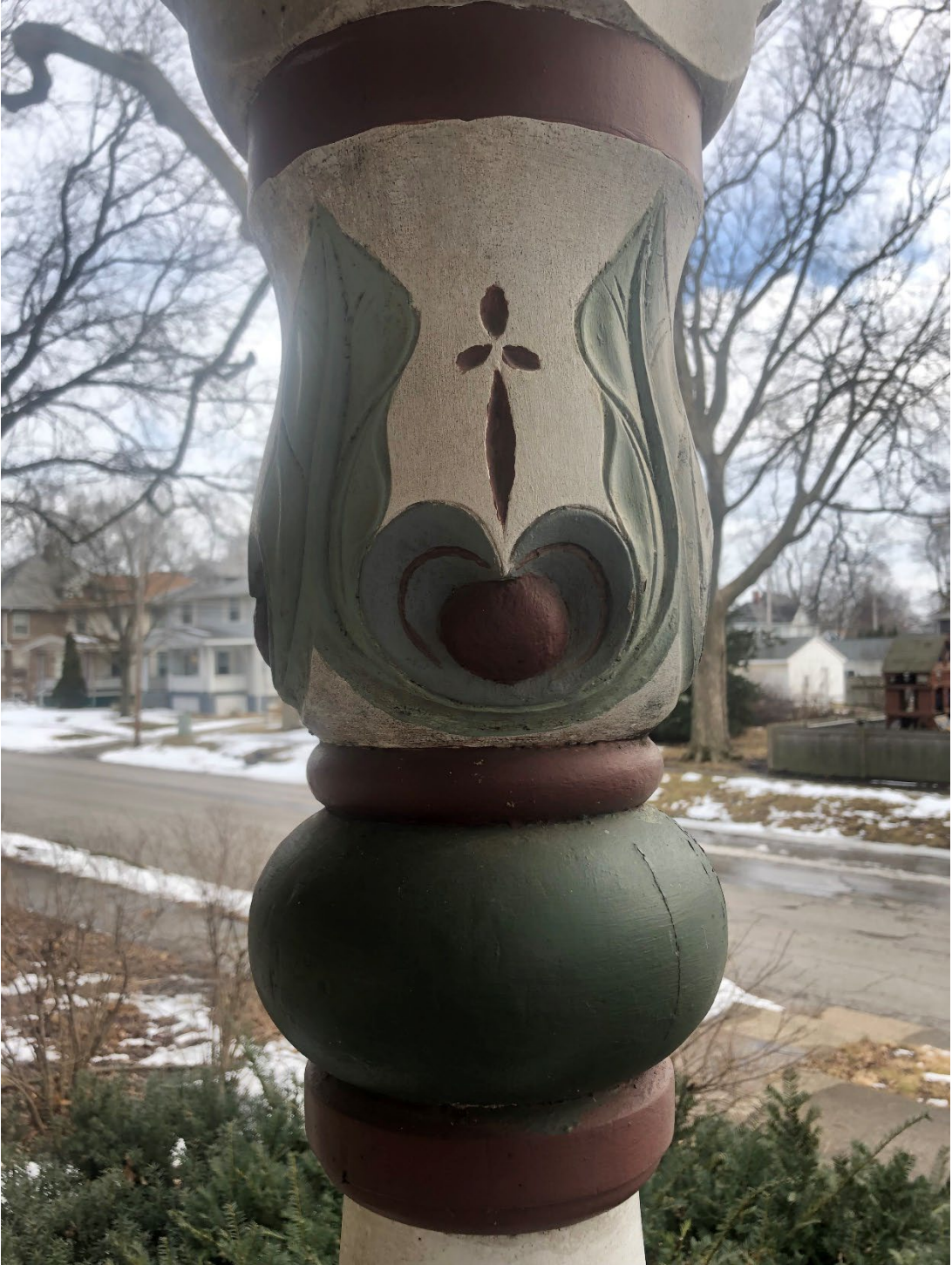
Detail of one of the porch columns.
