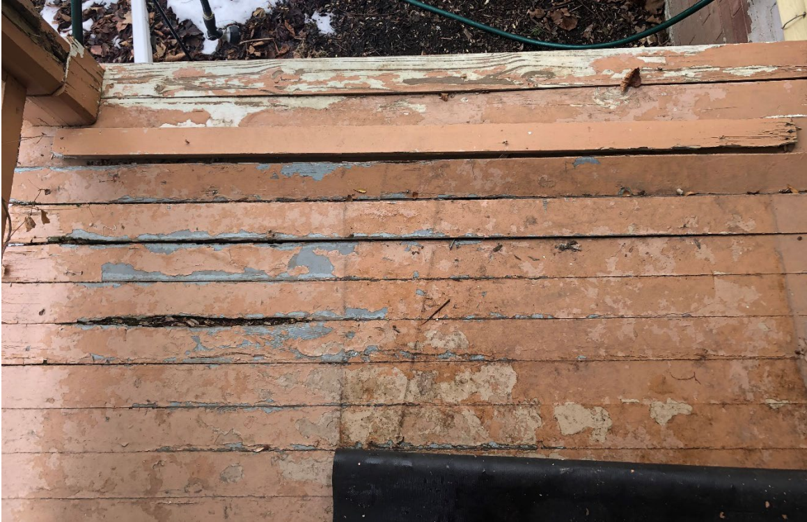
Wear and buckling to the deck boards.
