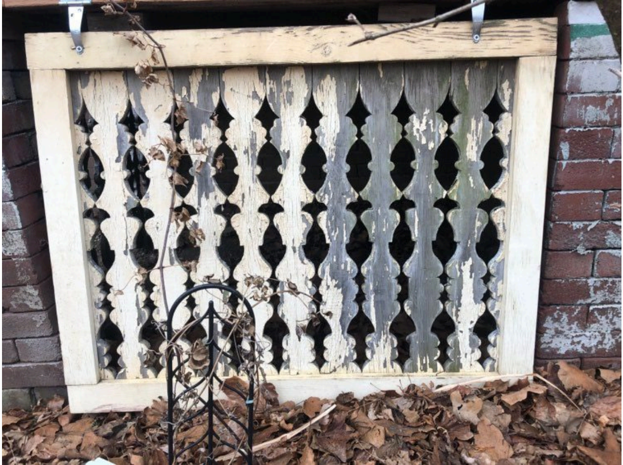
One of the remnants of the original porch skirting which used to decorate both the front and back porches and can be seen in two of the photos of the main application.
