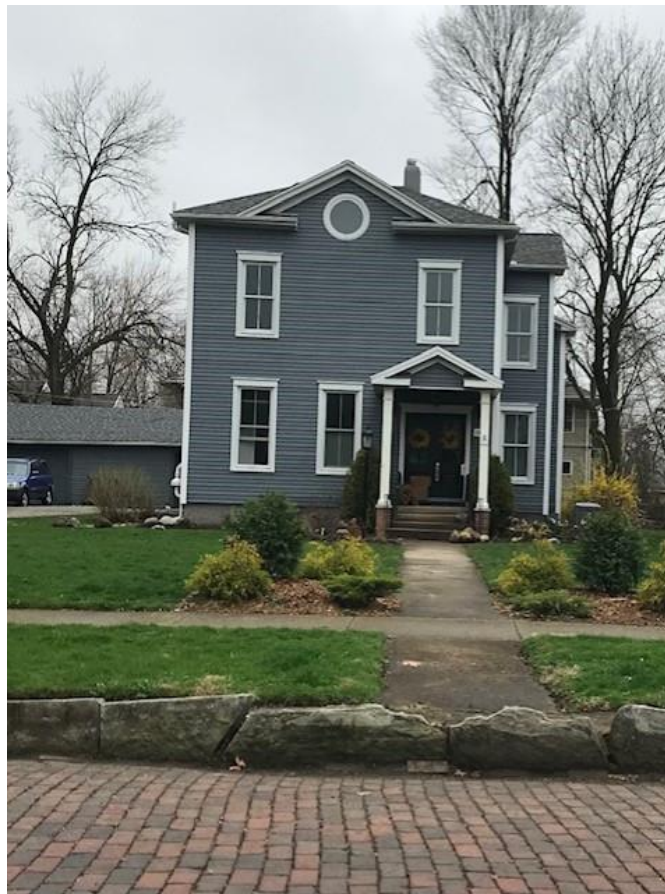
Above: The subject property at 1009 E Jefferson Street
