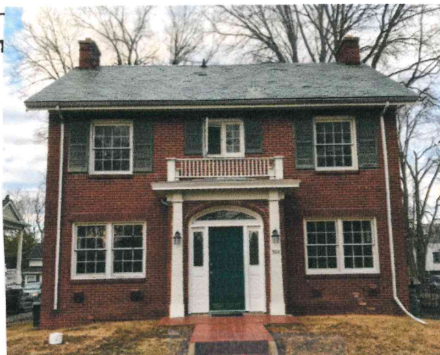
Picture of restored walkway
