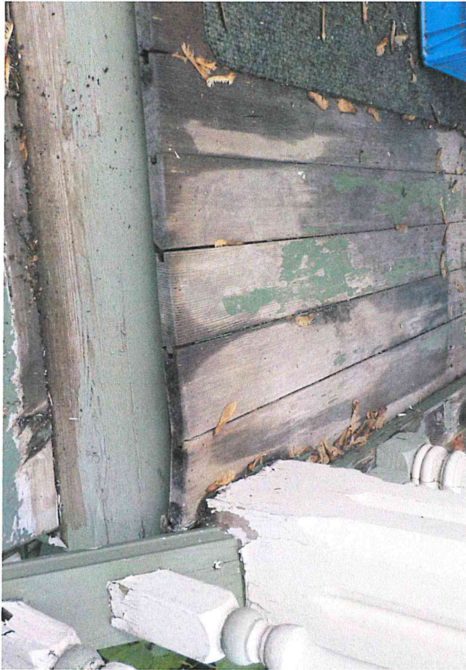
porch floor + spindles
