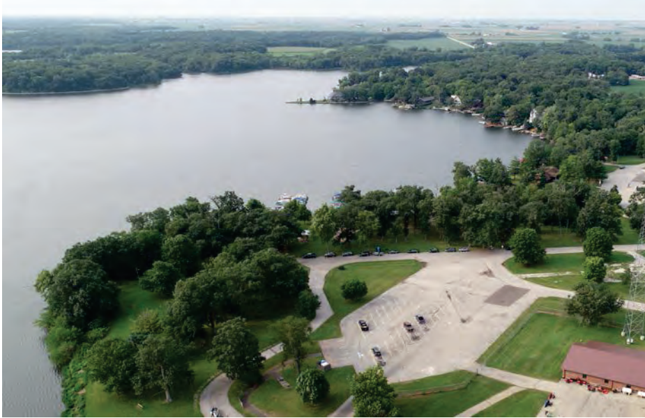
Lake Bloomington Facing South from WTP
