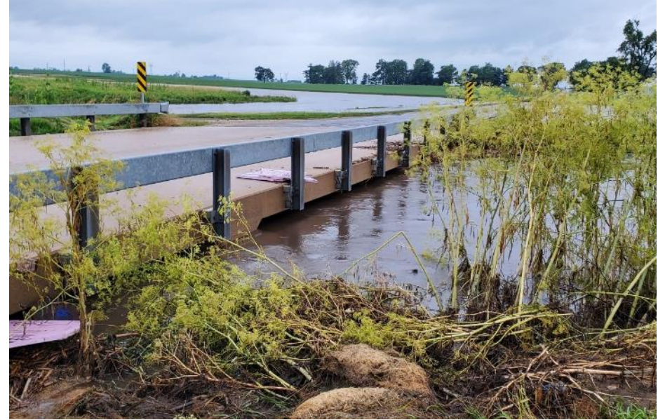
2100 East Bridge near The Grove
