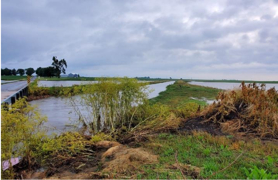
2100 East Bridge near The Grove
