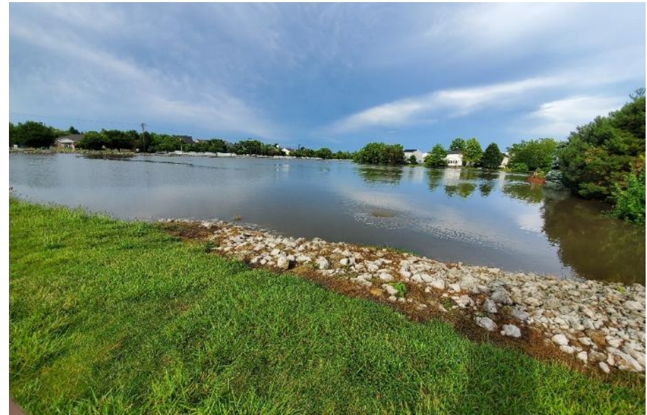
GE Rd near Airport Rd
