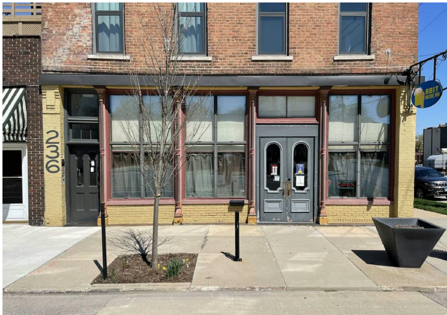
Above: The subject property at 236 E. Front Street
