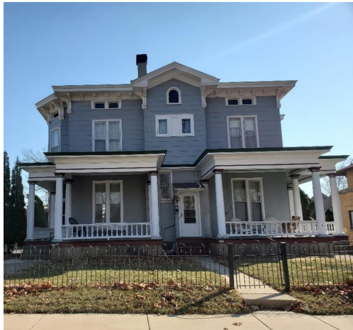
Above: The subject property at 319 E Chestnut Street.
