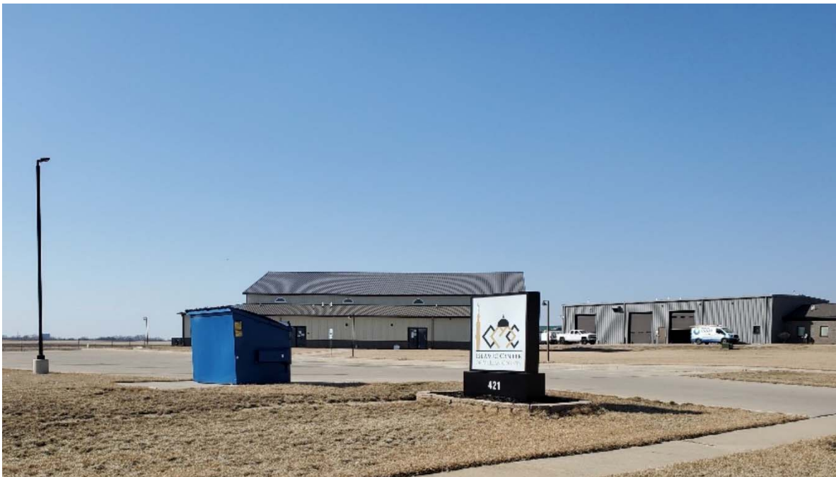
The existing site
