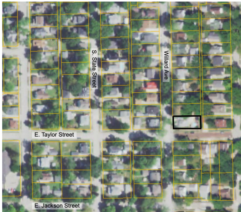
Figure 1: An aerial view of subject property, 220 Willard Avenue (outlined in black)
