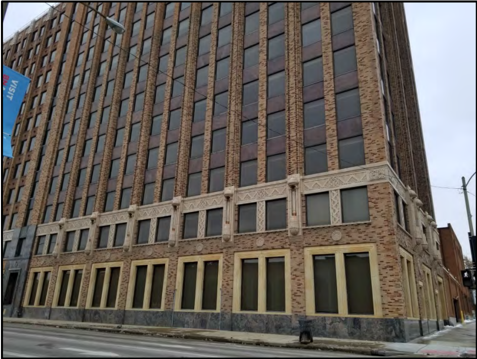
Figure 7 Northern portion of east elevation.
