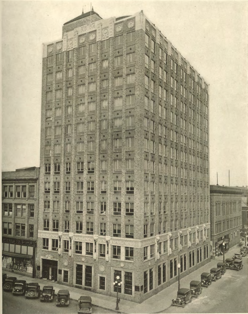
OFFICE BUILDING FOR THE STATE FARM INSURANCE COMPANIES, BLOOMINGTON, ILLINOIS
