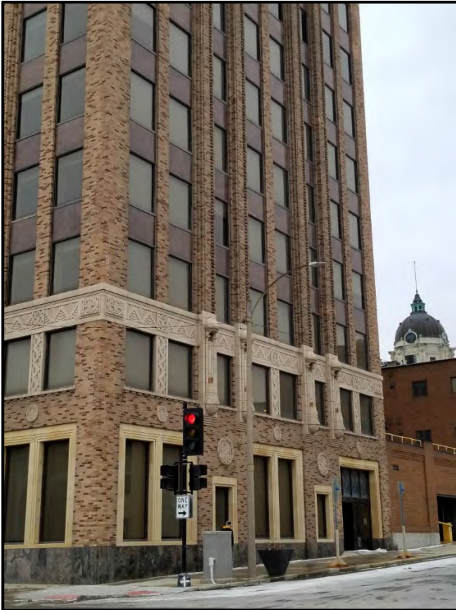
Figure 9 North elevation of the State Farm building.
