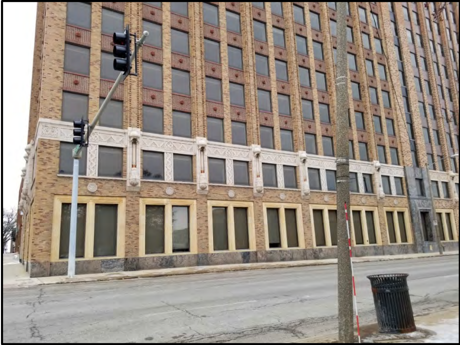
Figure 5 South portion of east elevation.
