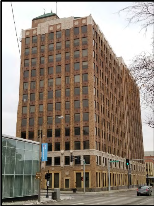
Figure 1 South and east elevations of the subject property, 112 E. Washington.
