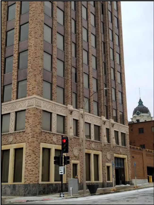
Figure 9 North elevation of the State Farm building.
