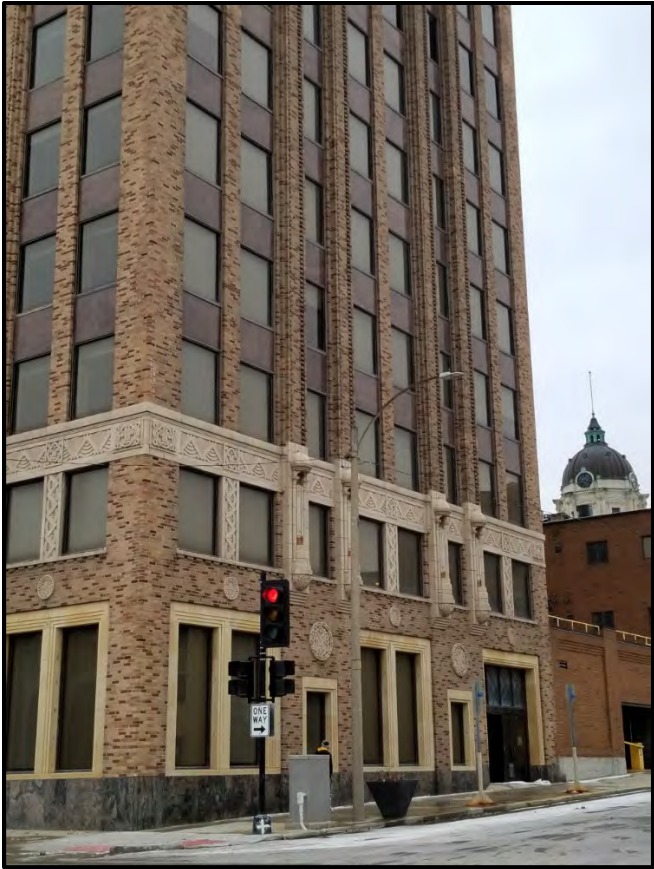
Figure 9 North elevation of the State Farm building.
