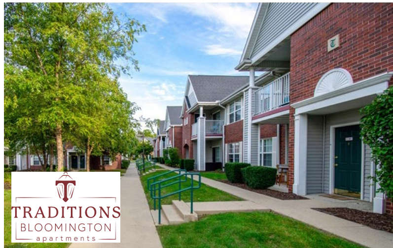
Figure 13: Traditions Bloomington Apartments Side Exterior
