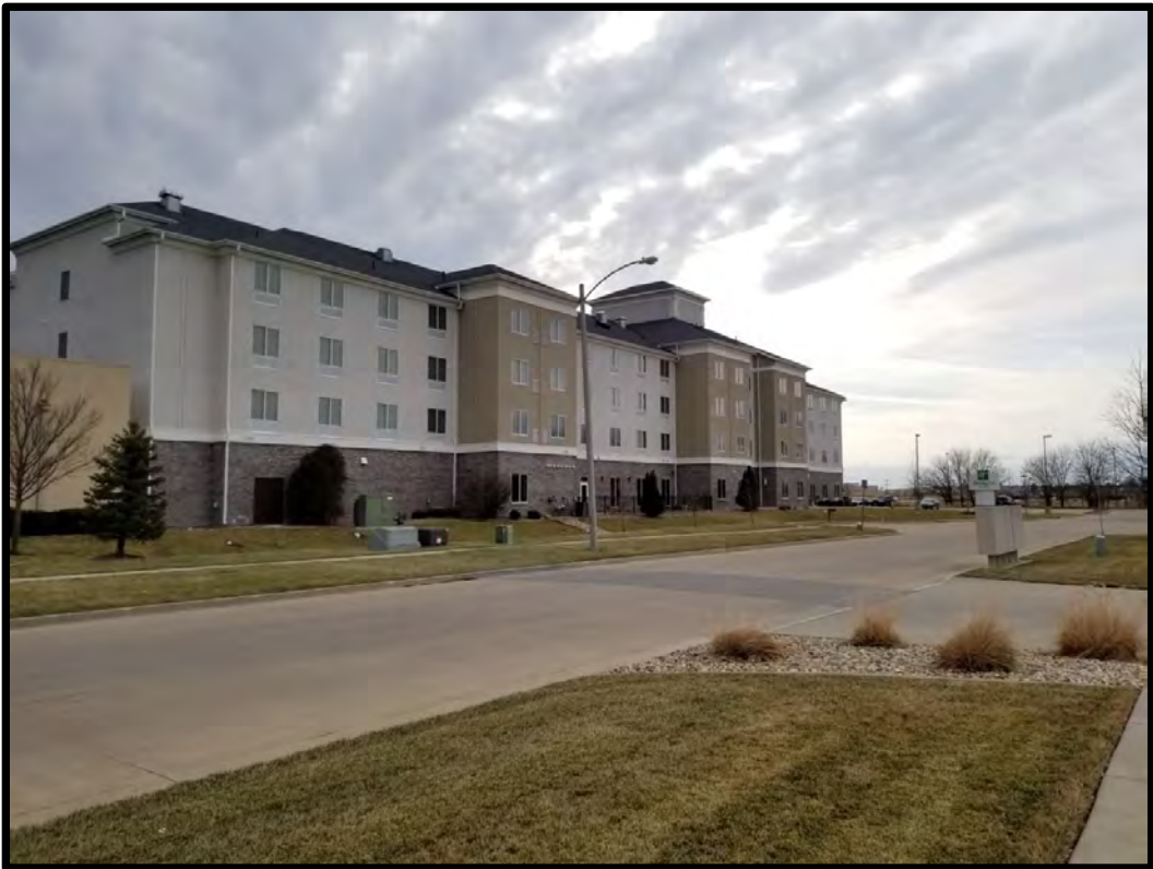
Figure 5 The rear elevation of Holiday Inn from Gerig Drive facing E. Empire Street.
