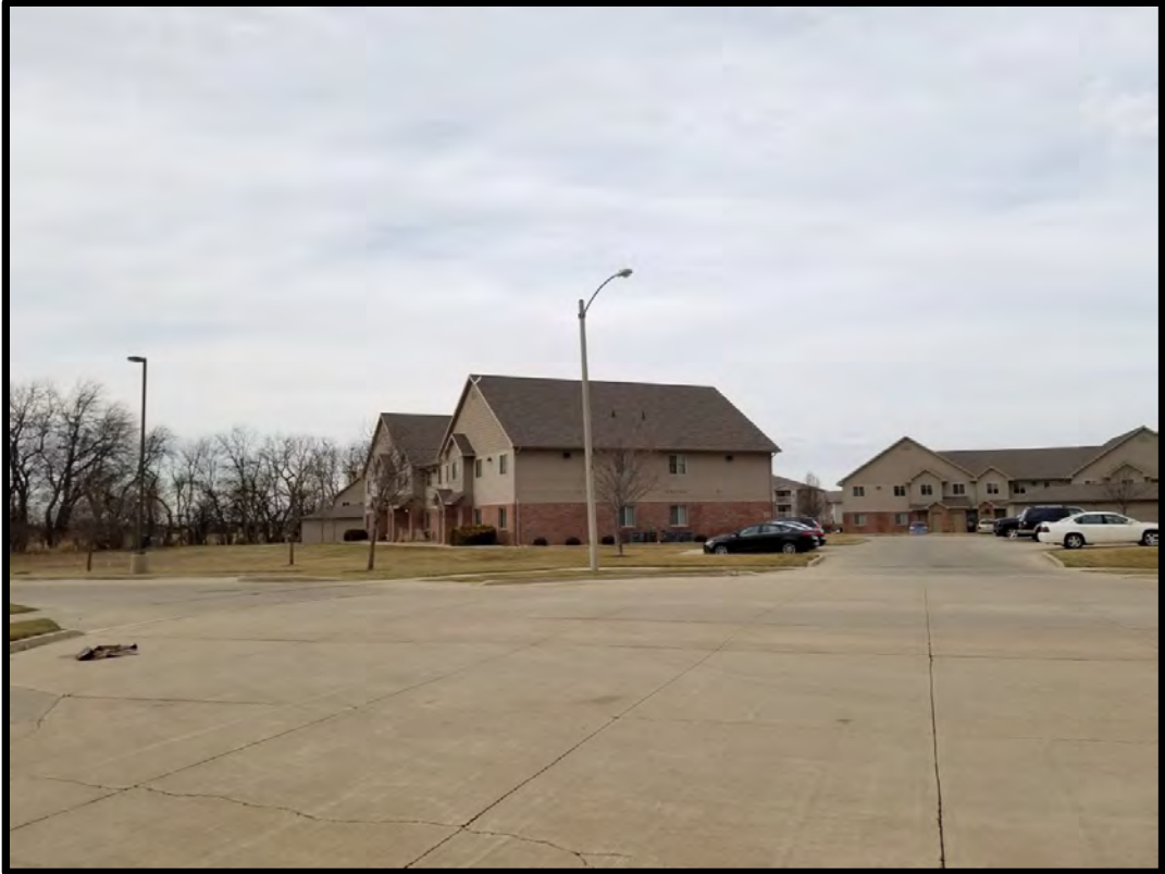
Figure 6 Multi-family residences at 3204 Gerig Drive.
