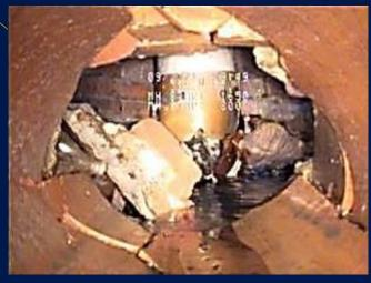
399 cracking near manhole, structural problems within manhole
